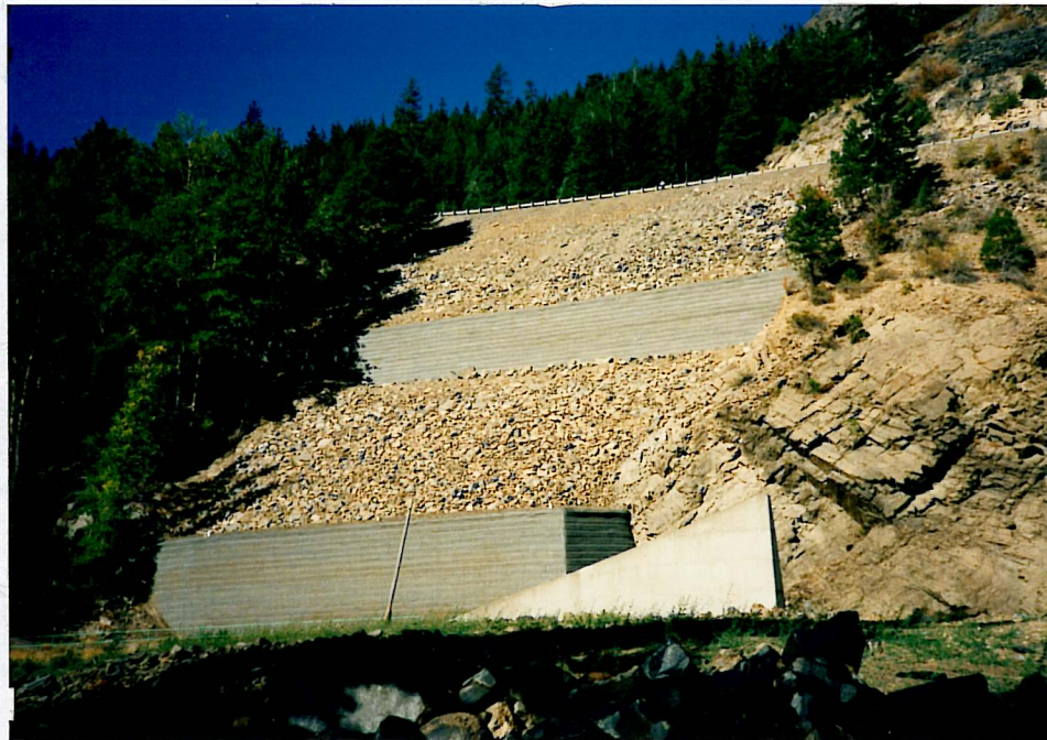
Tieton Dam Spillway Welded Wire Walls constructed by North Central Construction
