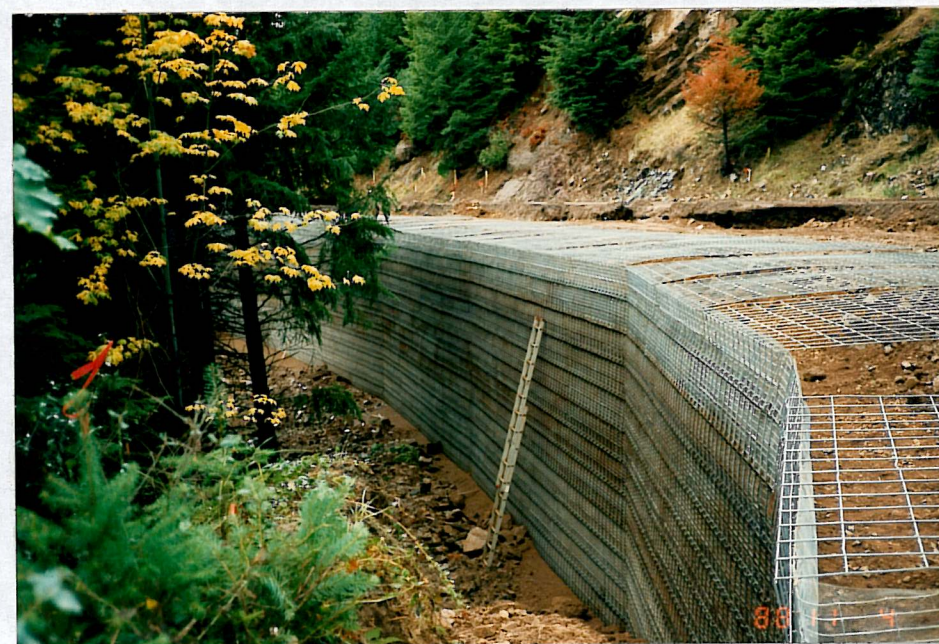
Various Welded Wire Wall in Washington, Utah, Arizona & Oregon
