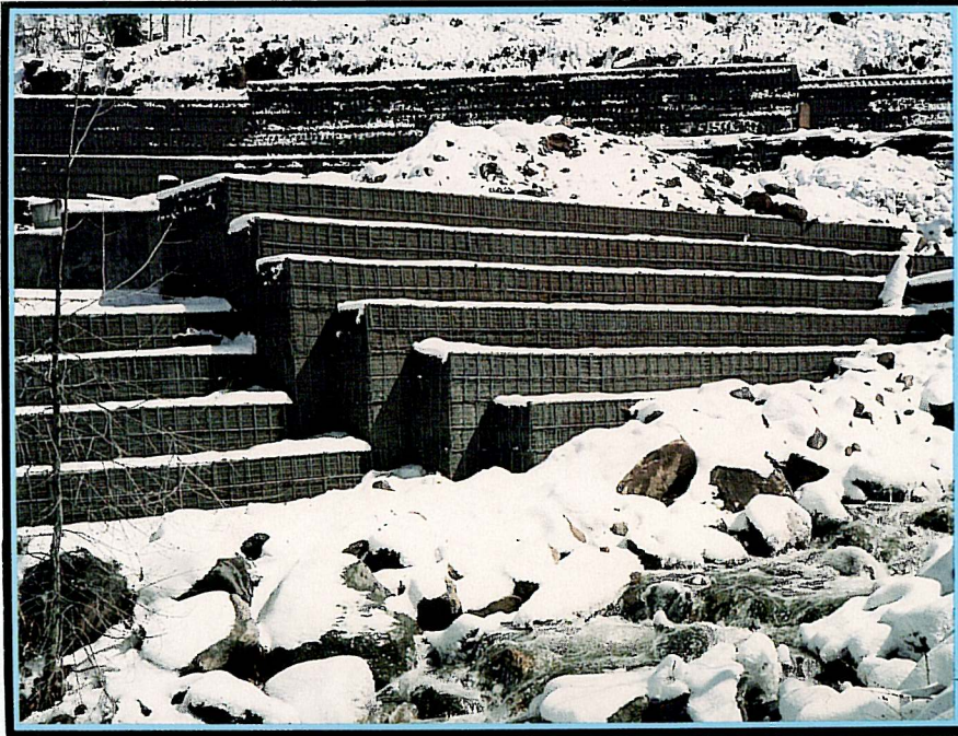
↑ WWW - TELLURIDE, CO. Private Project. Contr.: Baker Const. & Final Touch Const.
