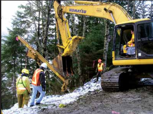
Vibro Percussion Sled on an Excavator
