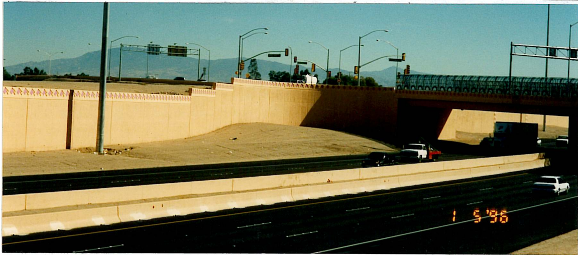
MIRACLE MILE TRAFFIC INTERCHANGE Eureka Reinforced Soil with CIP Face (42,224 Sq. Ft.) Interstate 10, Tucson, Arizona Arizona Department of Transportation Contractor: Hunter Contracting Company Engineer: ADOT & MacIntosh Engineering & Development May/June 1994
