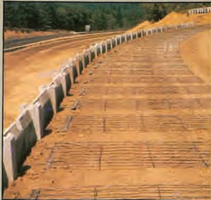
Mechanically Stabilized Embankment, bar mats in position.
