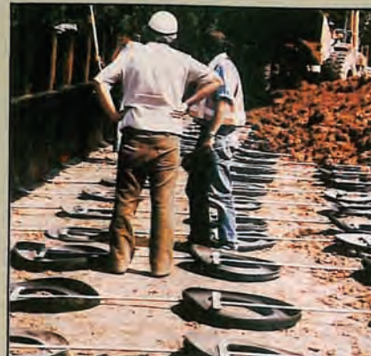
Recycling of non-biodegradable tire sidewalls in construction of "Tire Anchored Timber Wall."
