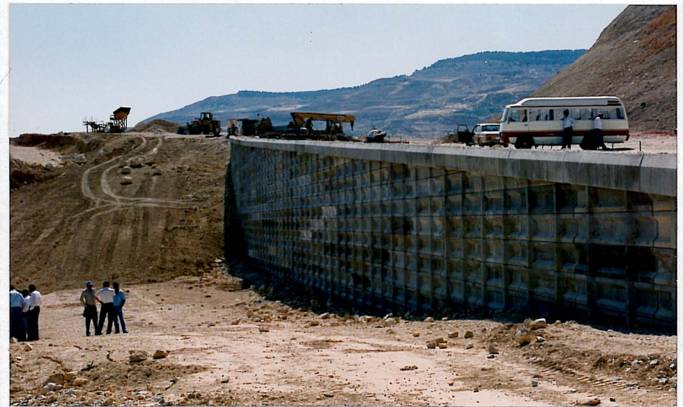
Dead Sea Highway, Amman, Jordan Jordanian Ministry of Public Works, Summer 1990 Reinforced Soil Embankment
