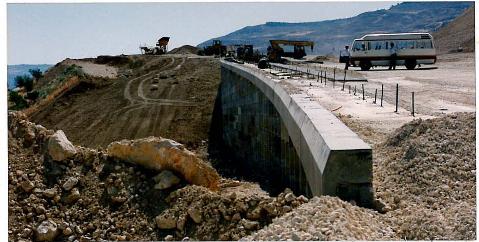
Dead Sea Highway, Amman, Jordan Jordanian Ministry of Public Works, Summer 1990 Reinforced Soil Embankment
