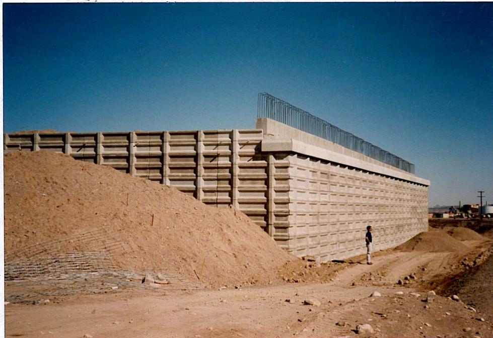
Reinforced Soil Embankment (Shadow Panel) NEVADA DEPARTMENT OF TRANSPORTATION Reno, NV
