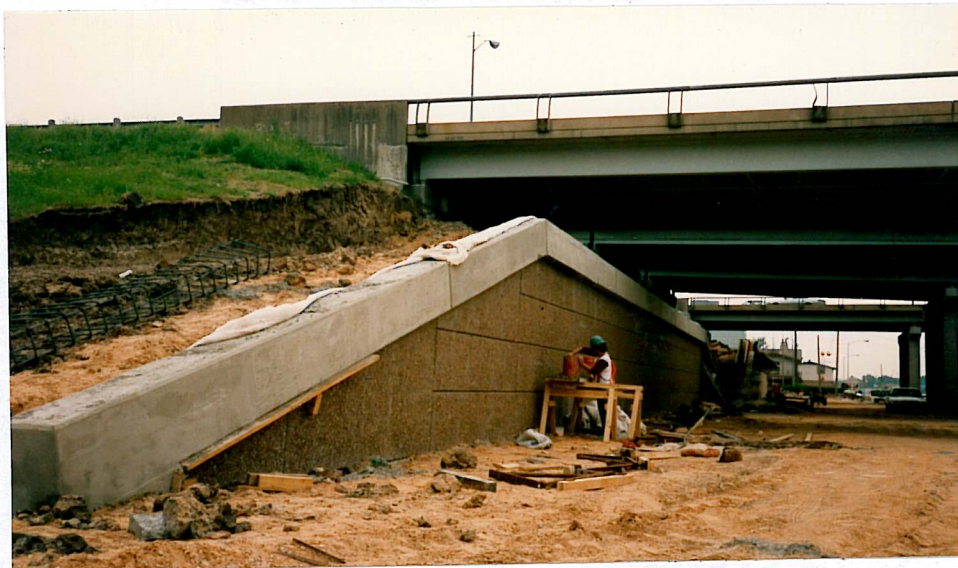
Reinforced Soil Embankment (R.S.E.) Smooth Face Panel w/Exposed Aggregate Houston, TX Contractor: Granite Construction
