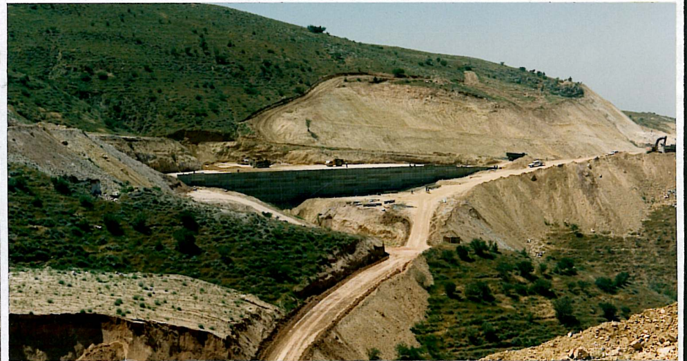
Reinforced Soil Embankment-Shadow Panel Dead Sea Highway, Amman, Jordan Jordanian Ministry of Public Works, Summer 1990
