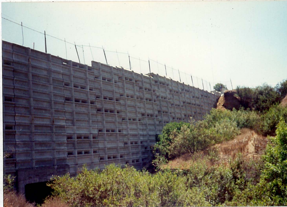
California Seabreeze - Costa Mesa Reinforced Soil Embankment with random planter panels constructed by Baker Construction & Van Dyk Engineering 714/744-1129
