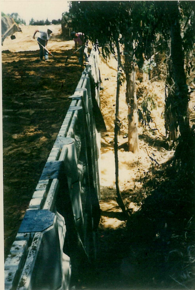
California Seabreeze - Costa Mesa Reinforced Soil Embankment with random planter panels constructed by Baker Construction & Van Dyk Engineering 714/744-1129
