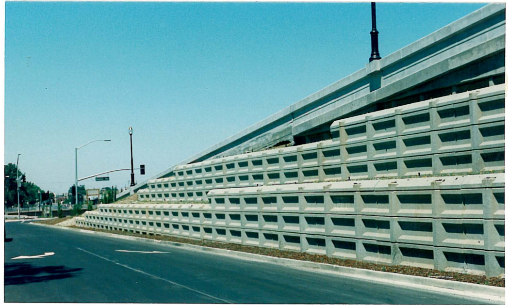
RAILROAD AVENUE R.S.E. Shadow Panel Retaining Wall City of Pittsburg, California Contractor: R.M.Harris Co. Engineer: DeLeuw, Cather and SHN & Assoc. Summer 1987 6,975 Sq. Ft.
