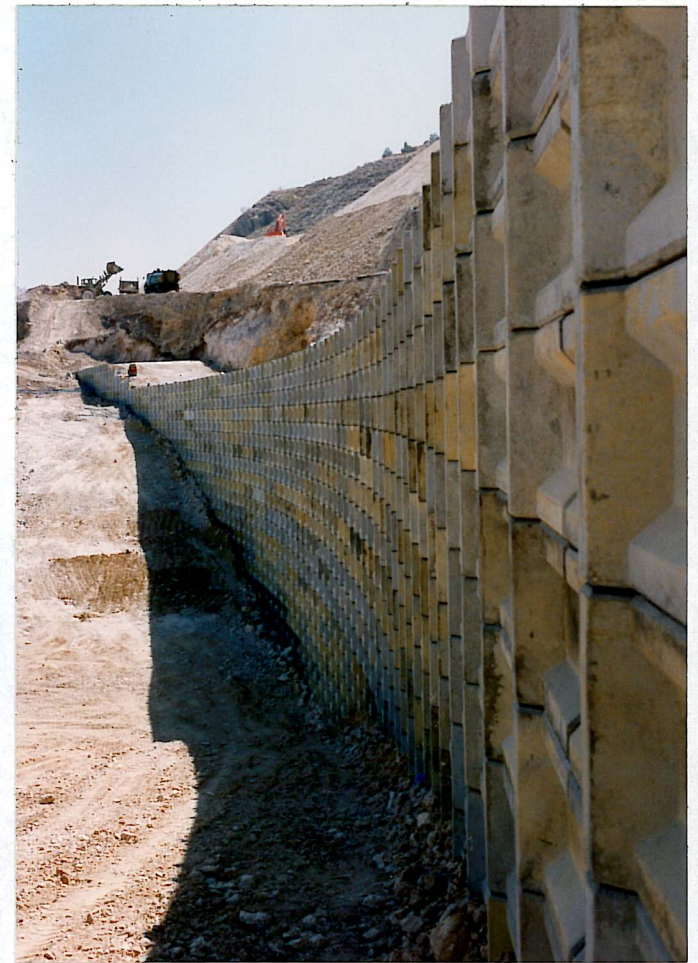
Dead Sea Highway Amman, Jordan Jordanian Ministry of Public Works Hudhud Shand Ltd. Summer 1990 Reinforced Soil Embankment
