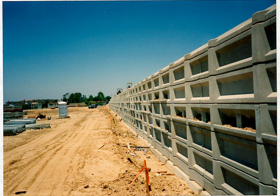
California Seabreeze - Costa Mesa Reinforced Soil Embankment with random planter panels constructed by Baker Construction & Van Dyk Engineering 714/744-1129
