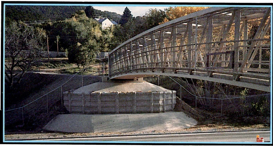
→ RSE - EXPOSED AGGREGATE - MESCALERO, NM. NM State Hwy. Dept. Contr.: C.S. McCrossan.
