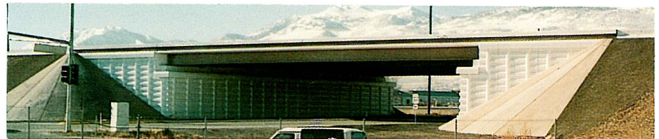
U.S. 395 - RENO R.S.E. Shadow Panel Retaining Wall Reno, Nevada Contractor: Helms Construction Engineer: Nevada D.O.T. and SHN & Assoc. Summer 1988 14,136 Sq. Ft.
