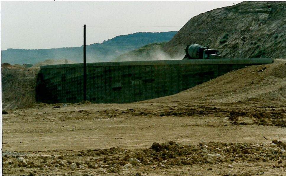
Reinforced Soil Embankment-Shadow Panel Dead Sea Highway, Amman, Jordan Jordanian Ministry of Public Works, Summer 1990
