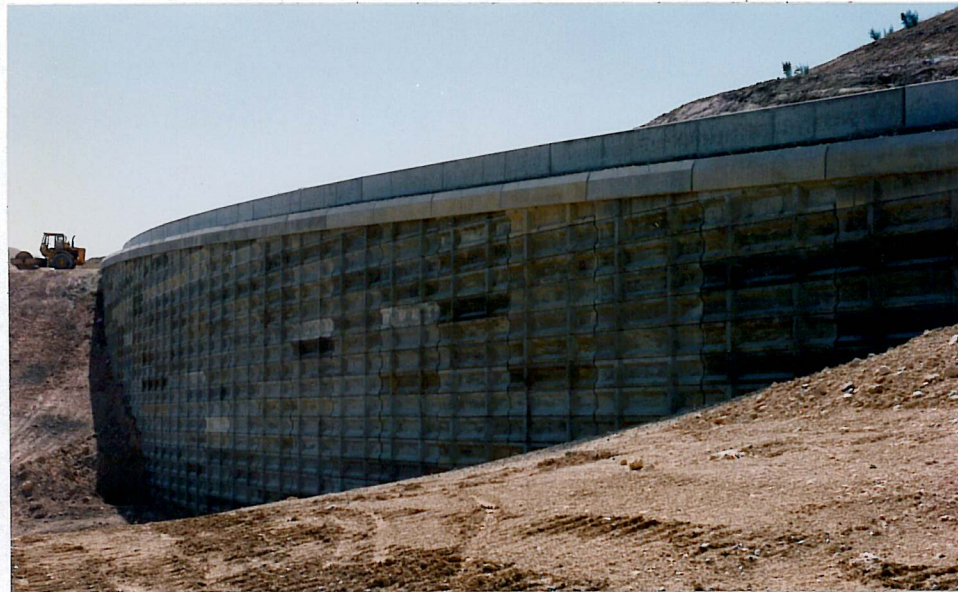
Dead Sea Highway, Amman, Jordan Jordanian Ministry of Public Works, Summer 1990 Reinforced Soil Embankment
