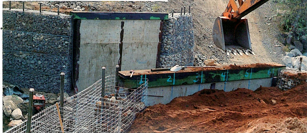
GRISWOLD CREEK, CALIFORNIA Constructed by Fiberboard Corporation
